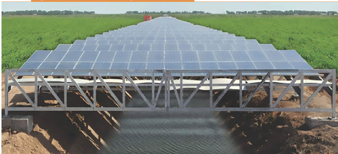
Figure 57 · Solar Panels Over Irrigation Canals in India
